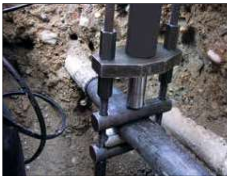
The cylinder/cross bar group can be detached from the clamp to leave it in compressed mode, the compression operation can be repeated in another point of the pipe with another clamp.
