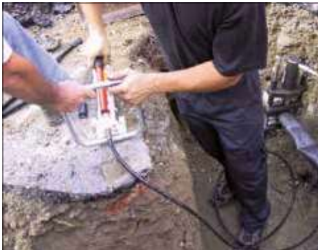
Pumping operation for pipe compressing
